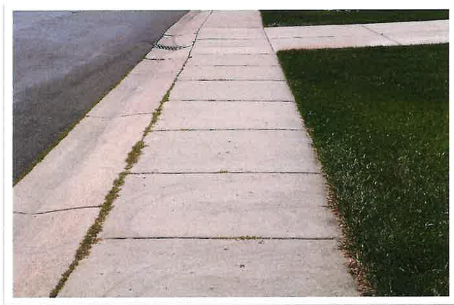
Photograph 2: Typical view of concrete sidewalk
