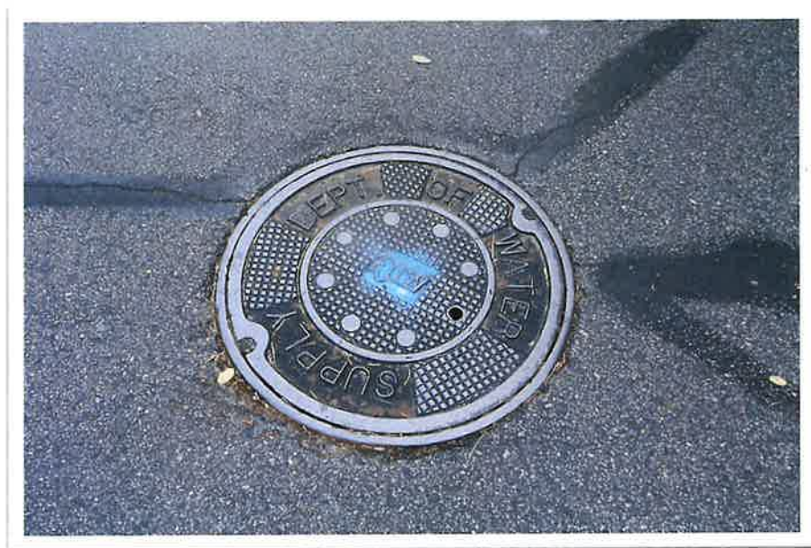
Photograph 7: Typical view of manhole
