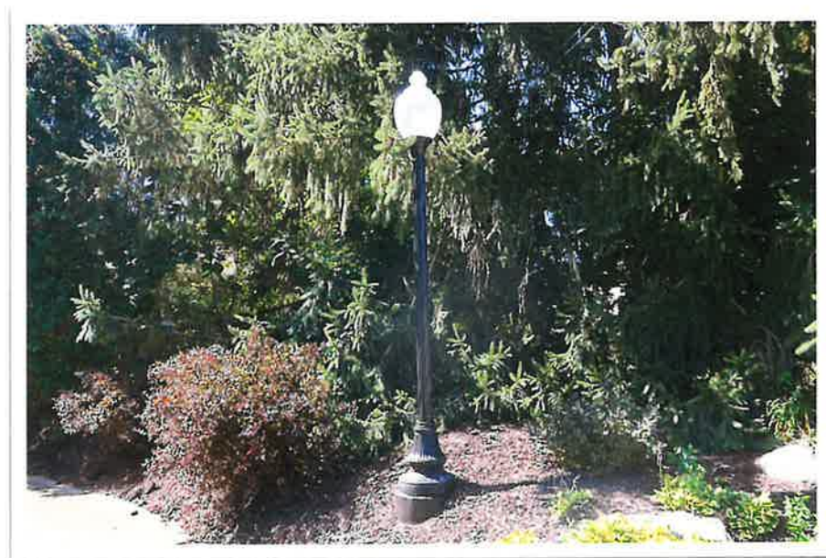
Photograph 8: Typical view of pole light
